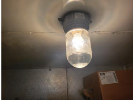
Light fixtures in both the walk-in cooler and freezer have accumulated condensation inside the lenses due to deterioration of the sealant around ceiling penetration and the interior of the electrical conduits.
