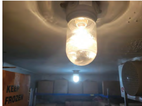
Light fixtures in both the walk-in cooler and freezer have accumulated condensation inside the lenses due to deterioration of the sealant around ceiling penetration and the interior of the electrical conduits.
