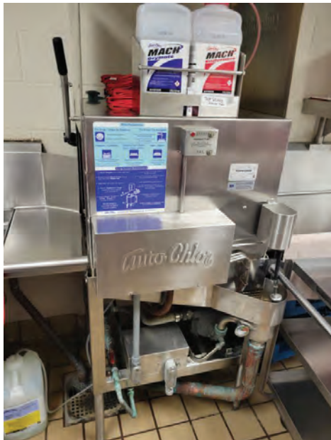
A ventless high temperature dishmachine is recommended to assist with the drying of the washing items.
