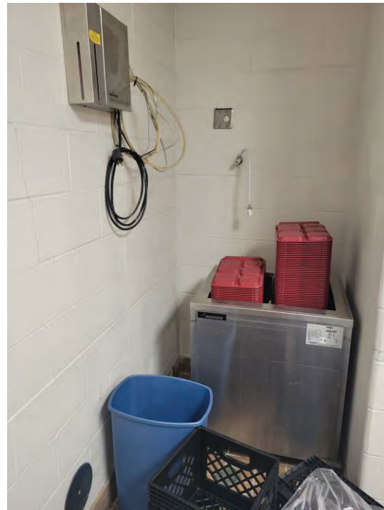
Recommend installing shelving in unused space for ice machine at the back of the serving area for disposable serviceware or ale carte items.
