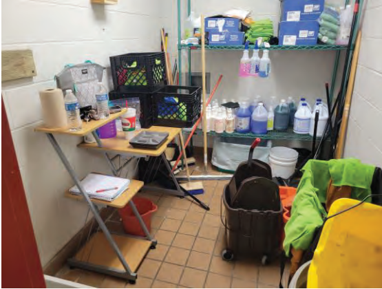
Additional storage shelving and the installation of a washer and dryer in the utility closet is recommended.
